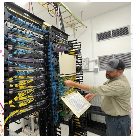
ABOVE: Our fiber foreman patching an Active Ethernet (AE) service at the POP, ensuring consistent connectivity for our customers.
