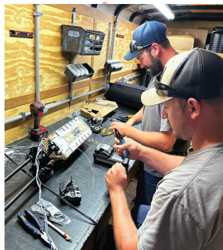
LEFT: Precision up close: A splicer in the bucket carefully working on the drop at the NAP, ensuring every connection is flawless.
